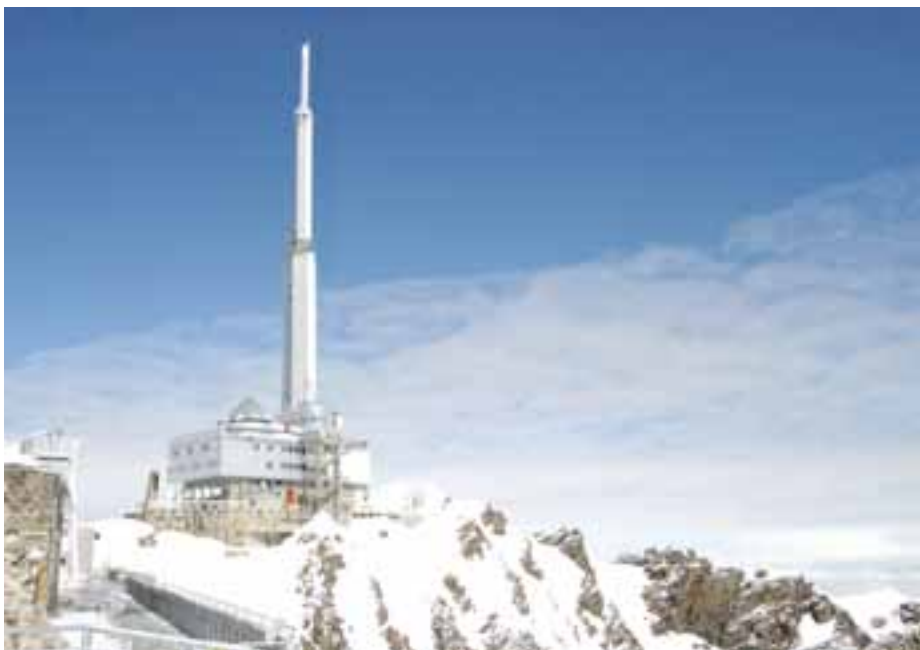
Lightning Protection Group at the Pic du Midi, close to Bagnères de Bigorre in the south west of France
